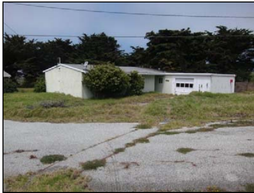
South and East Elevations
